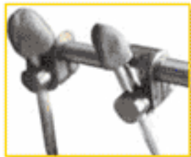
Protection of Cut Ends of Pins
